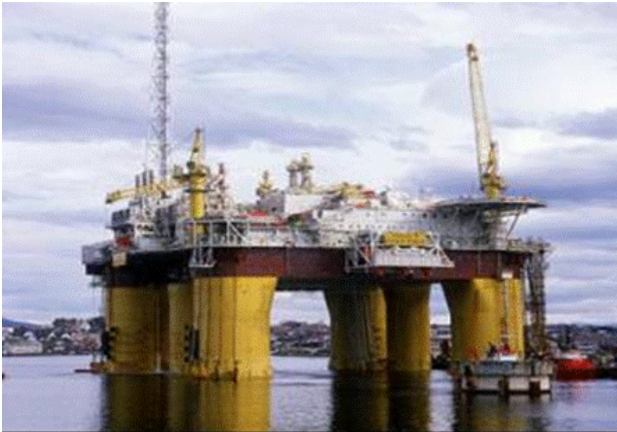
Figure 2 Offshore platform with module for living quarters
